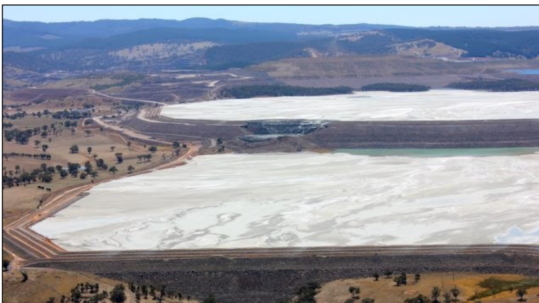
Figure 3 The tailings dam failure at Cadia mine in Australia. Image from Newcrest.
